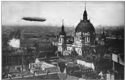
Keeping watch over Berlin, the men on this airship can see the whole city and its suburbs. The view is west from the City Hall toward the Parliament building
